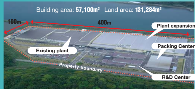
Status of new construction and expansion at No.2 Kyushu Plant
